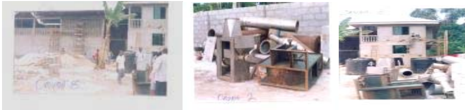
Mobilizing of machines to the Omuma site
